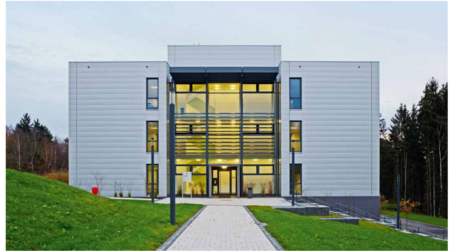
The recently completed building for the new Max Planck Department, a junior research group, an independent Max Planck Research Group, and the Flow Cytometry and Protein Diffusion & Interactions Unit.
